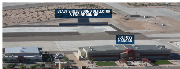
Blast shield sound deflector located adjacent the Joe Foss Hangar
