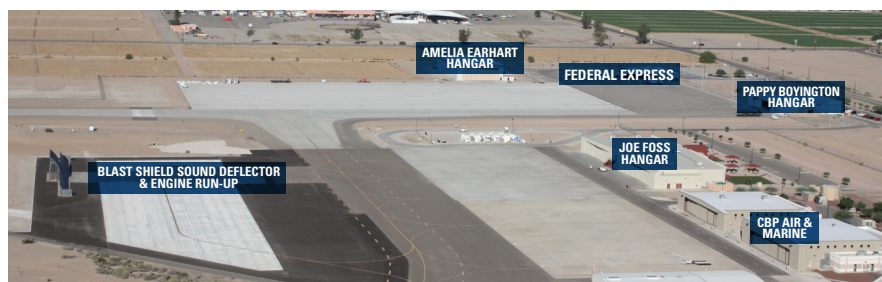
Aerial view depicting facilities blast shield sound deflector and engine run-up areas
